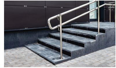
Staircases & its Metal railings
