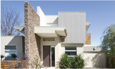
Vertical cladding of Stones
