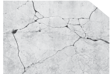
Thermal Cracks
